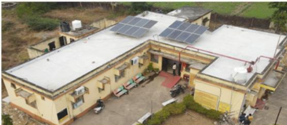
Plate: Primary Health Center, Village Nagardhan, Block Ramtake
