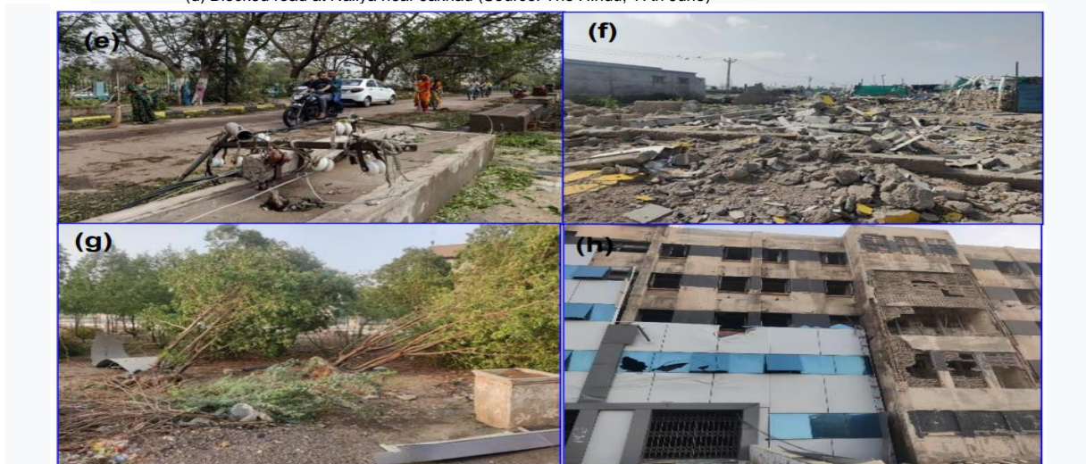
Plates: (e) Damaged electric poles in Kutch district (Source: PTI, 17th June) (f) Damage at Jakhau Port (g) Damaged trees at Kandla Port and (h) Damaged buildings at Kandla Port (Source: f to g Post Cyclone Survey team, IMD)
